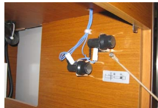
Battery support (System piezo) Access: beneath the oven
