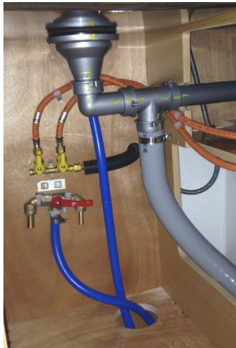
Gas supply valve Access: Under the sink
